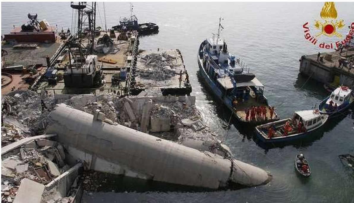
The Control Tower after the accident
